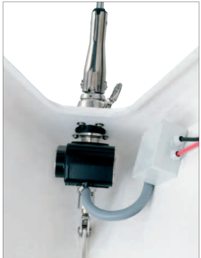
Installation of a Furlex 200TDE. The connection box is water-tight.
